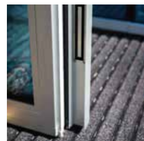
Concealed electromagnetic lock on the opening frame
