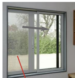
Mesh comes across the window on opening allowing good visibility but preventing the flow of contraband in or out of the window
