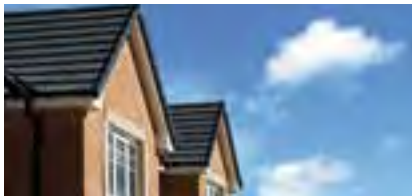
Fascias, soffits and guttering
