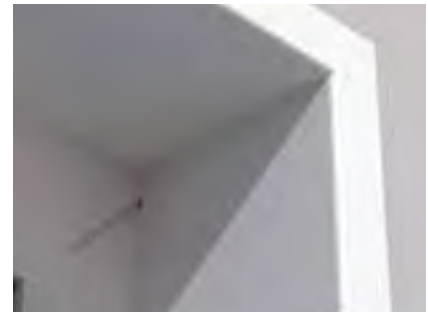
9mm capping board used as a reveal liner
